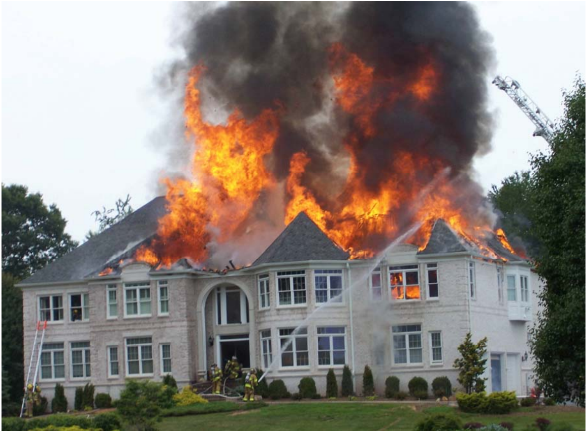
View from the street of the house prior to E434 exiting the structure.
