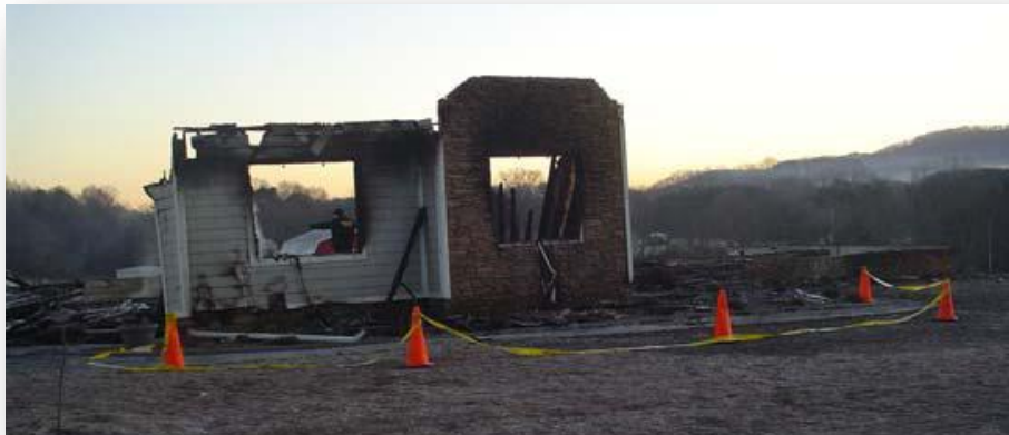
Image from the January 26, 2007, fire that claimed Volunteer Firefighter Shane Daughtee (NIOSH Report 2007-07)
