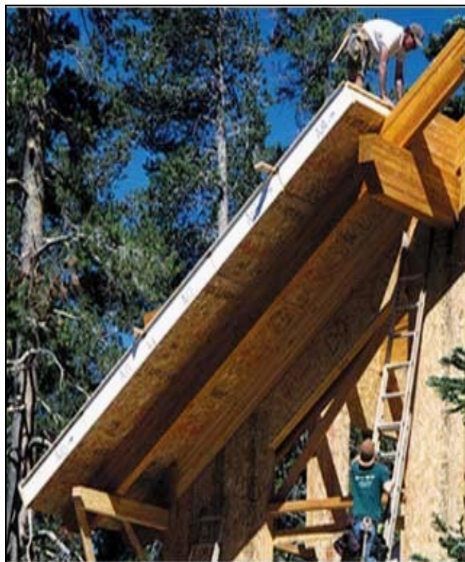
Figure 4 Structural Insulated Panel Roof Assembly
