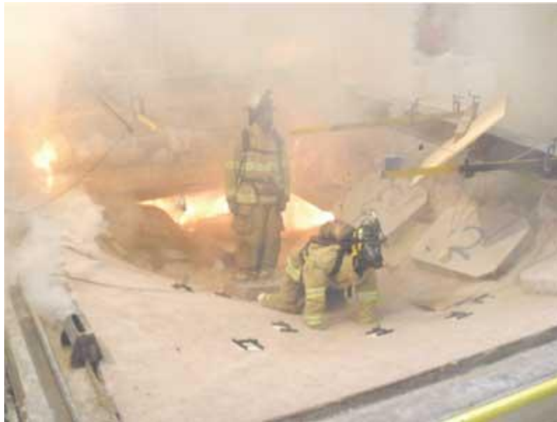
(5) A modern lightweight 12-inch wood I-joint floor—without ceiling. Collapse Time = 06:03. (5) The excessive floor deflections at the time of failure. (6) The condition of one of the surviving engineered I-joists after extinguishment.
