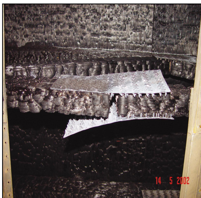
Figure 1: Metal Connector Plates After Fire Test
