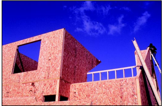
Figure 9 Wood Structural Insulated Panel (SIP) Installations
