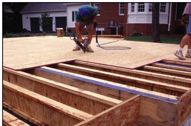
Figure 7 Single-Layer Floor Panel Installation
