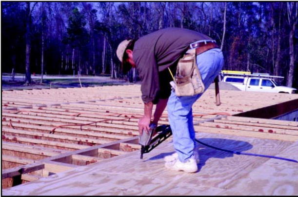
Figure 10b Floor Construction
