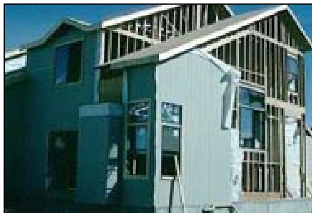
Figure 8a Siding Installation
