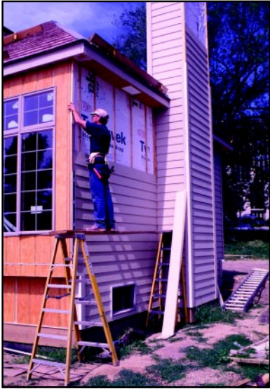
Figure 8b Siding Installation
